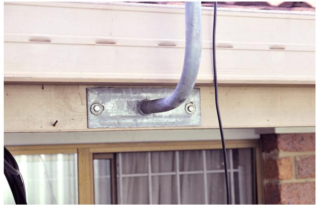
The author was going to weld a suitable mount together out of scrap steel, but cost of the steel and mucking around simply wasn't worth it. A ready made galvanised TV antenna mount is a much easier solution.
