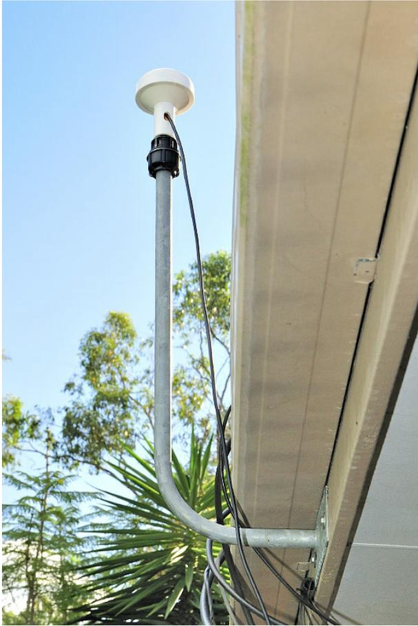
A TV antenna bargeboard mount is used, and these can be obtained for around \$20-\$25 new.
