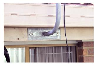
The author was going to weld a suitable mount together out of scrap steel, but cost of the steel and mucking around simply wasn't worth it. A ready made galvanised TV antenna mount is a much easier solution.
